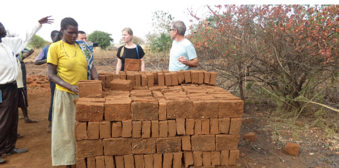
Bricks molded by women in Agago for Church building
